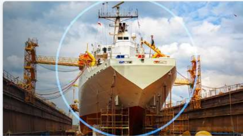
Challenge: Optimizing Shipyard Infrastructure
